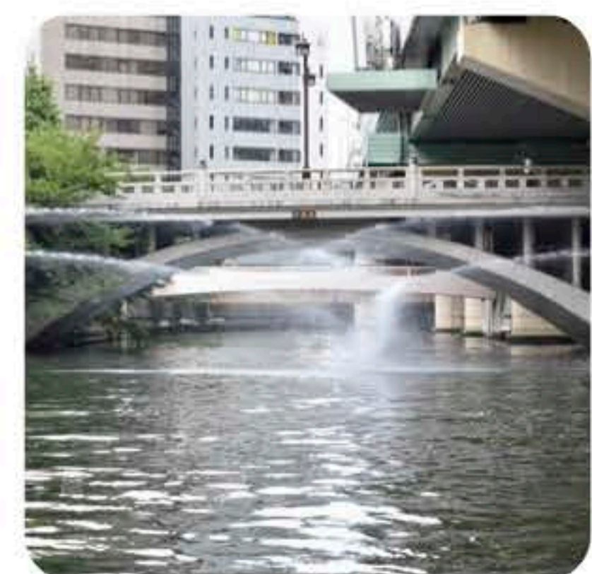
Regulating Gate of Higashi Yokobori-gawa
